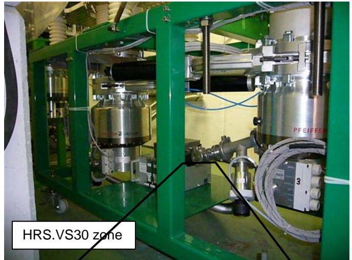
Leak-detection connection added on the TP at extraction side
